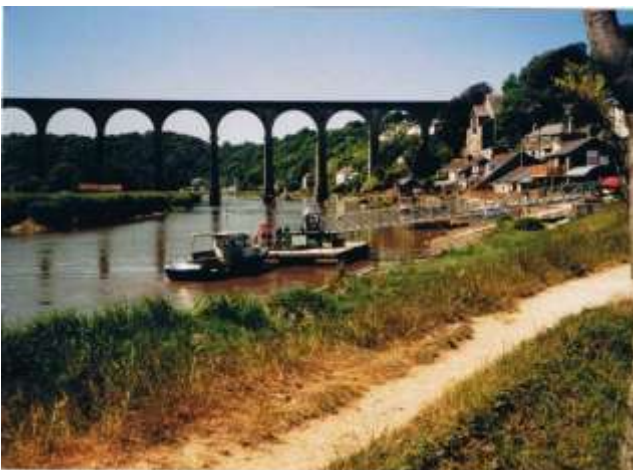
Calstock viaduct and the River Tamar
